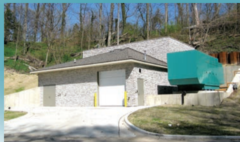
Raw Water Pump Station
