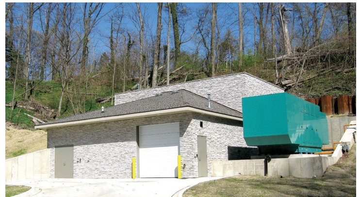
Benton Charter Township Raw Water Pump Station
