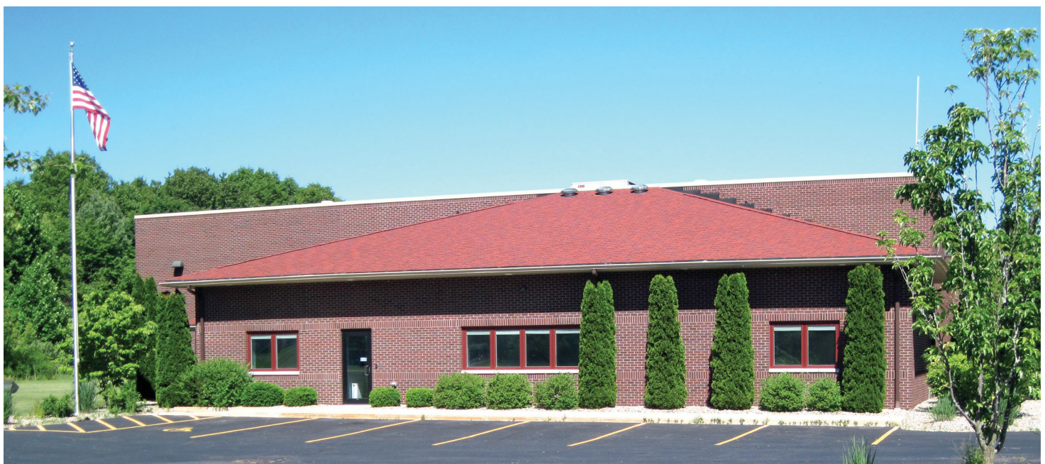
Benton Charter Township Water Treatment Plant
