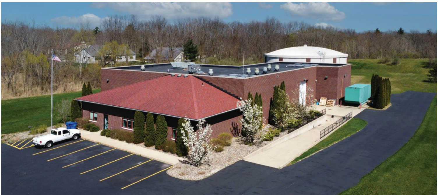
Benton Charter Township Water Treatment Plant
