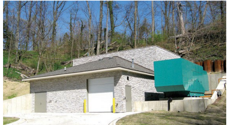
Benton Charter Township Raw Water Pump Station
