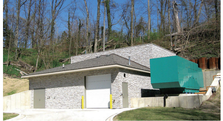
Benton Charter Township Raw Water Pump Station
