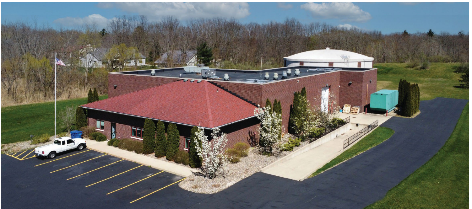
Benton Charter Township Water Treatment Plant
