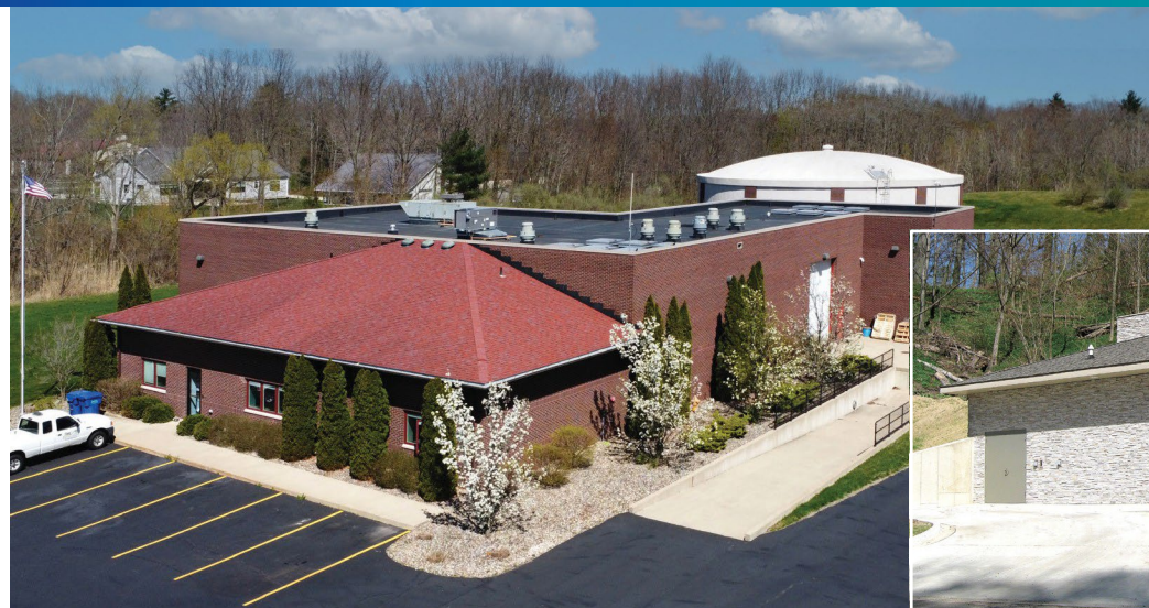
← Benton Charter Township Water Treatment Plant
