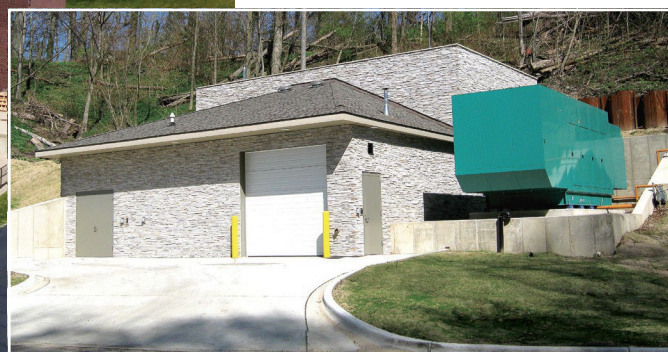
↓ Benton Charter Township Raw Water Pump Station
